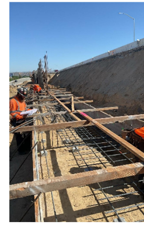
Retaining Wall 2809 Rebar Placement
