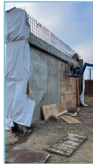
Stripping Forms Van Nuys Abutment 5
