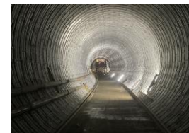
BL R5 Install of Liner Plate along Lasky Zone
