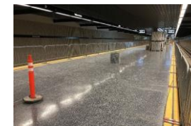
Wilshire/Fairfax Station: Platform View
