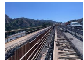
Gavin Canyon Bridge Right Formwork
