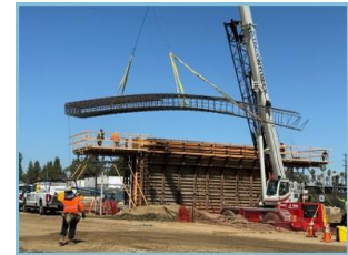
Setting Reinforcing Steel at Van Nuys Abutment 5
