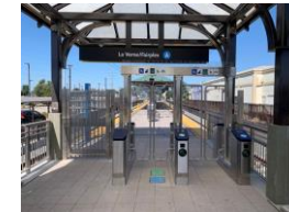
La Verne/Fairplex Station faregates installation near completion
