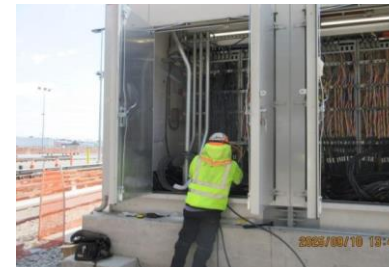
Train control cable installation at Bungalow B
