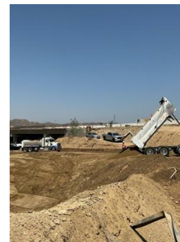
Embankment Fill at Rye Canyon
