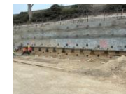
105WB-RW270 - Installing weepholes with geo-composite drain strips with meshing on row 4
