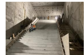
CCS Concourse Entrance Stair #3
