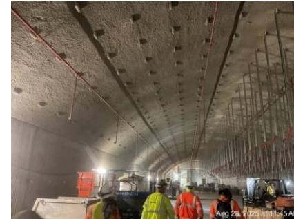
Westwood/UCLA Station: Installation of Overhead Fire Sprinklers on Concourse
