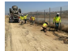
Fencing Install NB north of Castaic Creek
