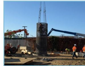
Setting Column Cage at Van Nuys Bent 2S
