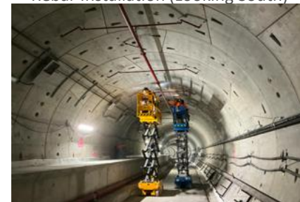
Tunnels: Tunnel Lighting Installation Reach 7 BR Tunnel
