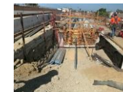
105WB-Yukon - Contractor preparing conduit to be installed on bridge
