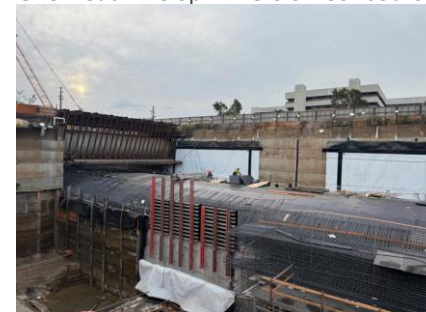
Westwood/VA Hospital Station: Roof Rebar Installation (Looking South)
