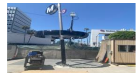
Wilshire/La Cienega Station: Station PIN Wire Work
