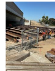
105WB-Dominguez Channel - Setting falsework beams
