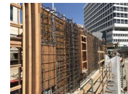
BDS Station Entry Portal Rebar and Formwork - Architectural Cast-in-Place Wall
