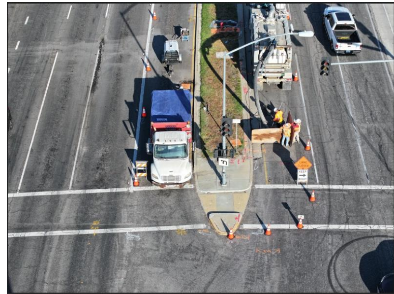
Potholing in Glendale
