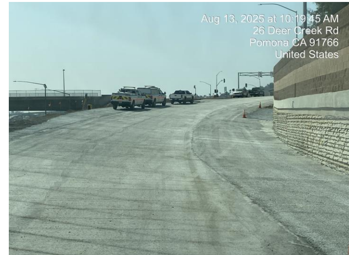
Realigned SB Rio Rancho off-ramp, LCB paving.
