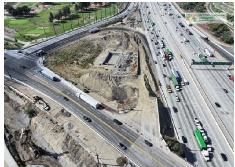
New SR-60 On and Off Ramps opened to traffic
