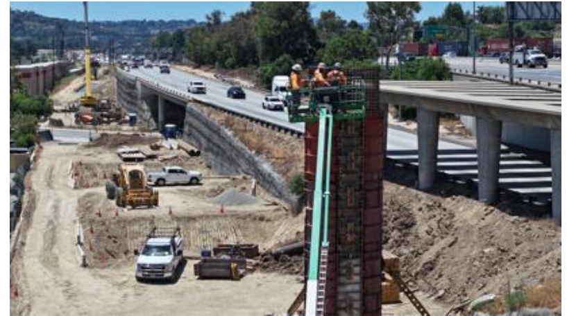
Construction of columns for EB SR-60 Bypass Bridge
