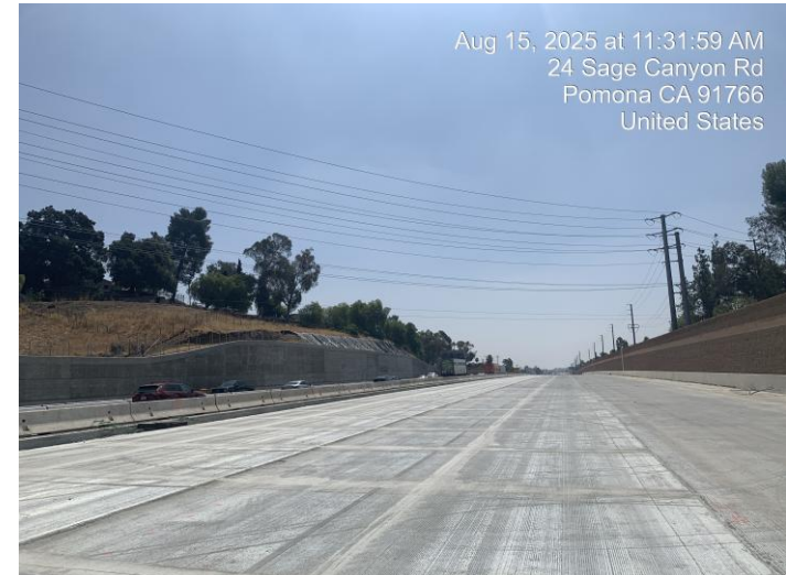
Stage 3, SB-71 paving.
