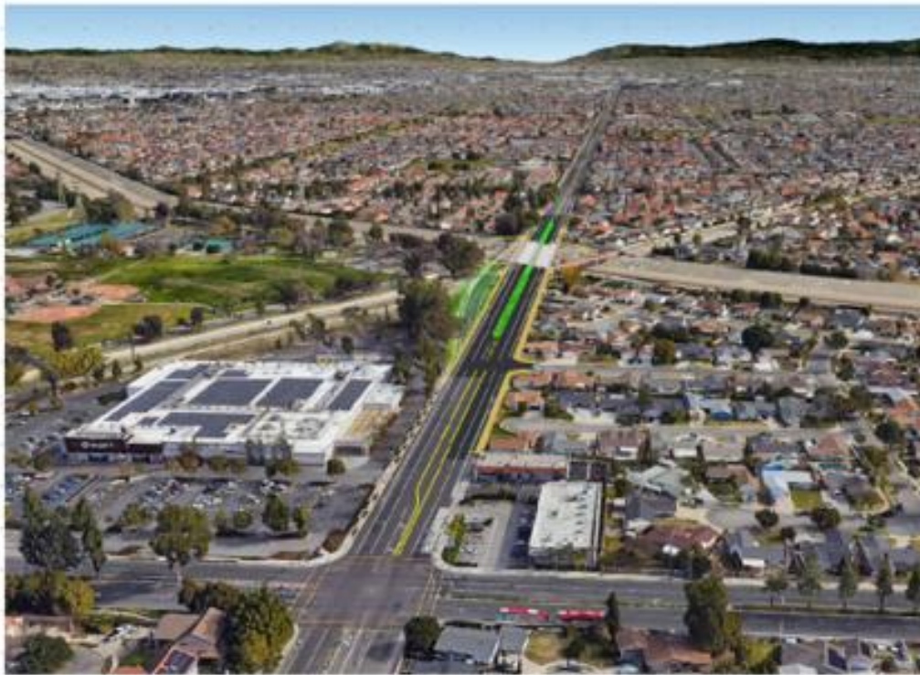
Del Amo Boulevard Project Overview Looking East
