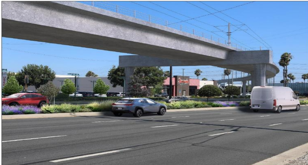
Figure 3.3-82. Simulation View, looking south/southeast from Hawthorne Boulevard near 186th Street towards Jerome's Furniture Store and Auto Dealerships (Draft EIR, 2023)
