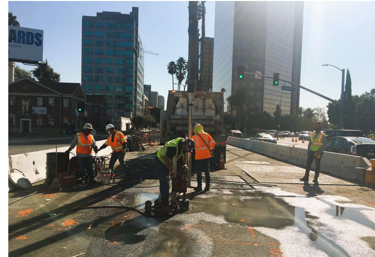
Potholing for Wilshire/San Vicente Tunnel Anomaly
