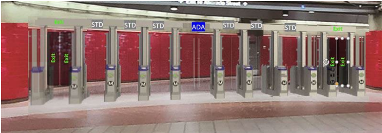
Proposed faregate array at Westlake/MacArthur Park, which uses taller faregates in lieu of emergency swing gates for egress, which had previously been misused over 25,000 times per week
