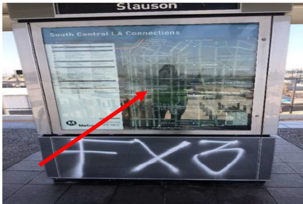
Slauson Station: 2024A-006 July 30, 2025 - Damaged Map Case
