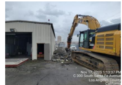
Legacy TPSS Demolition
