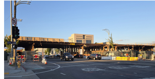
Falsework for Van Nuys Bridge
