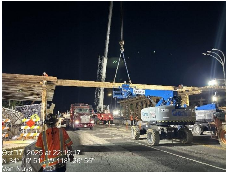
Setting Bents and Welding Stringers at Van Nuys
