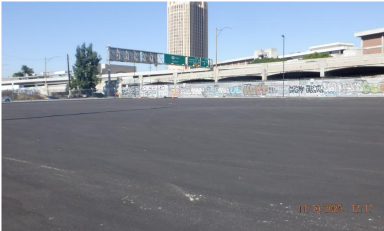
Building demolition & site paving complete (December 2025)
