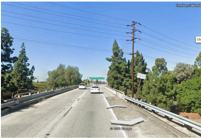
WB 91 to 605 Connector - Utilities Relocation at Studebaker
