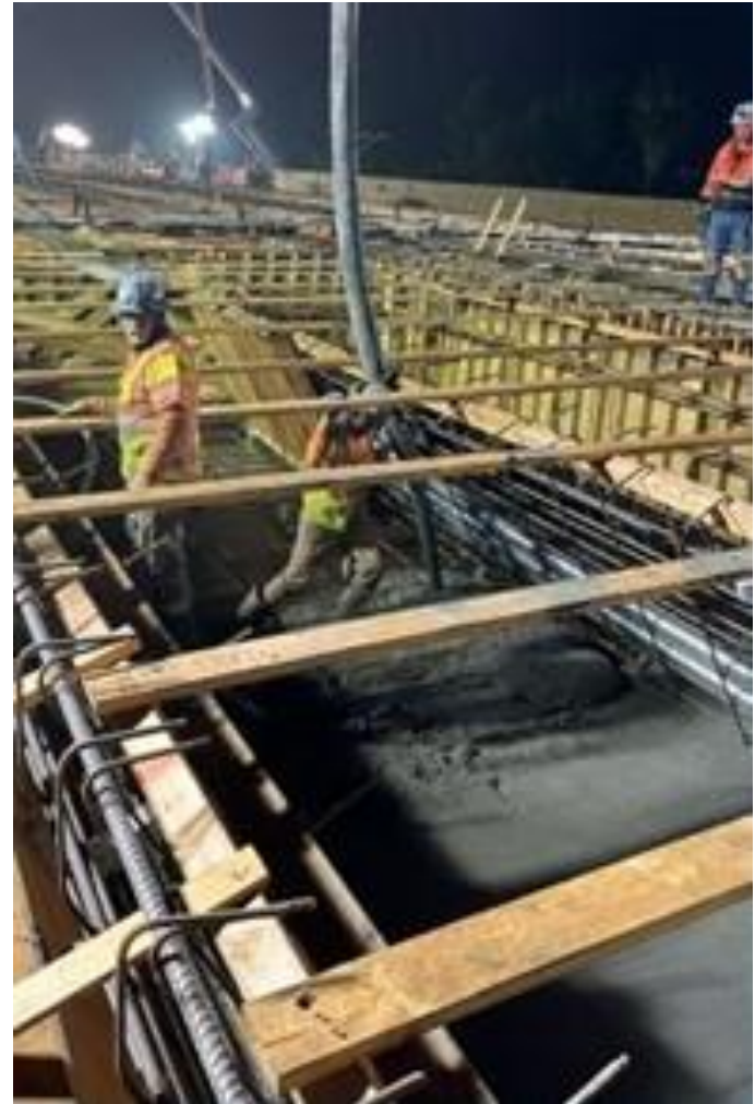
Concrete Placement for Van Nuys Bridge
