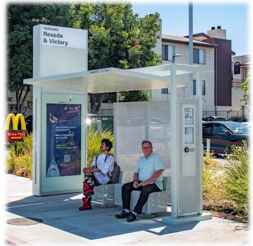
Bus shelter installed at Reseda and Victory
