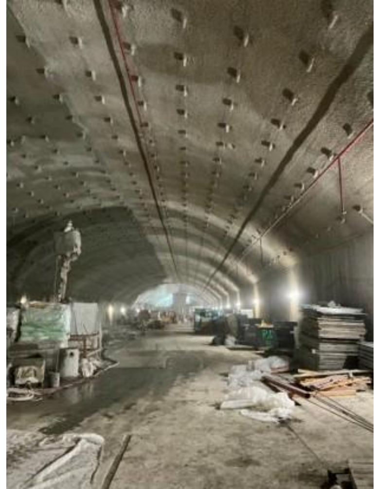
Westwood/VA Hospital Station Arched Roof
