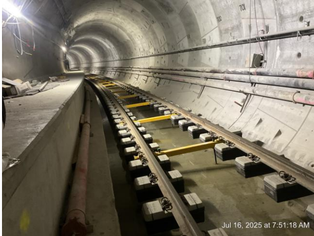
BR Tunnel Reach 5 Track Installation
