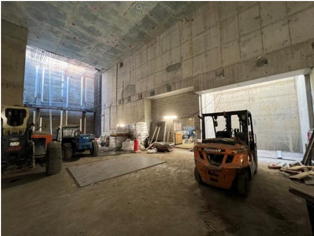
Westwood/UCLA Station Northeast Entrance Excavation
