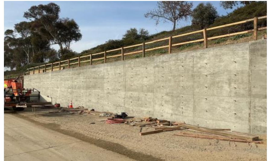
Stripping of forms from retaining wall
