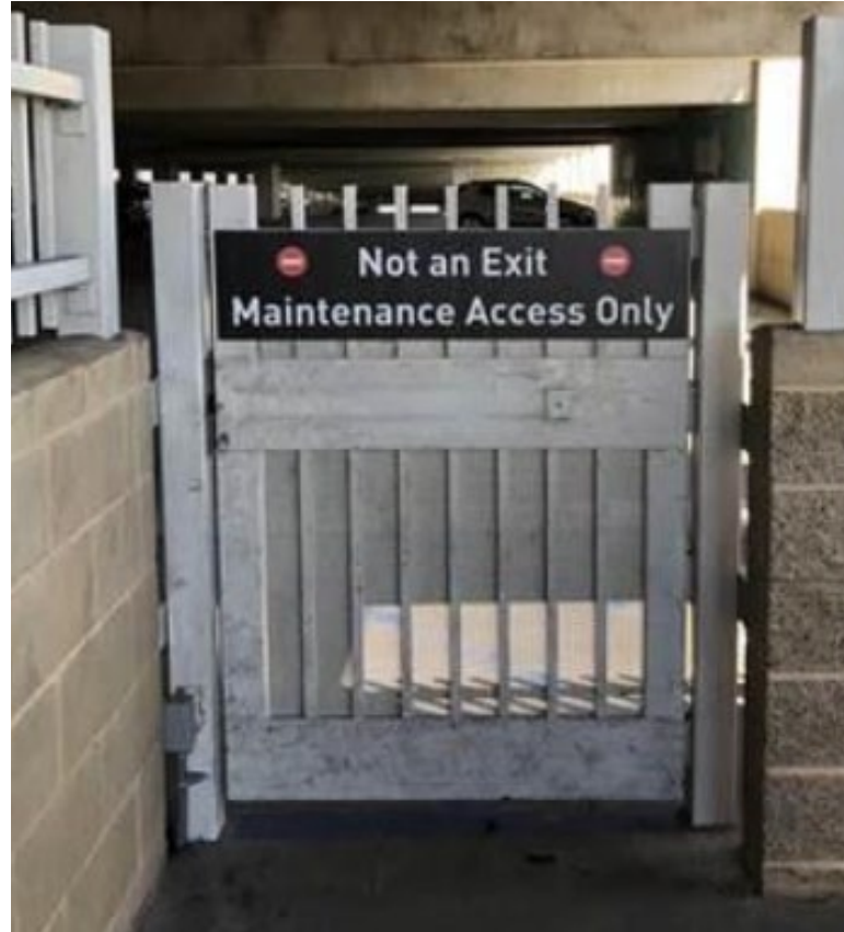
Before: Legacy ESG with easy access to the push bar for determined fare evaders
