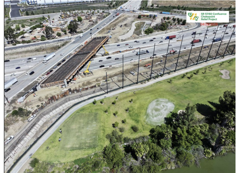
Placement of rebar and formwork at Grand Avenue bridge
