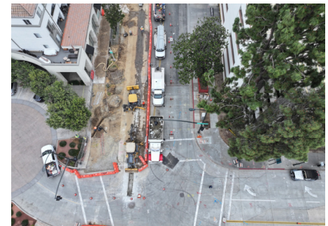
Holly and Arroyo Westbound Station Construction
