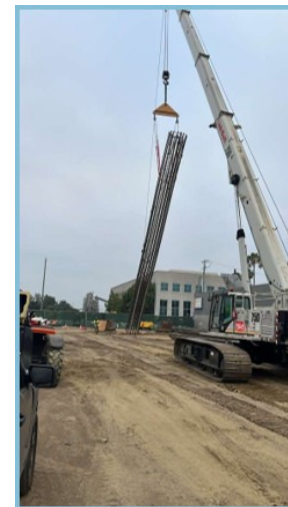
Setting Cages for CIDH Piles at Sepulveda
