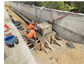
Drainage System 222 Installation
