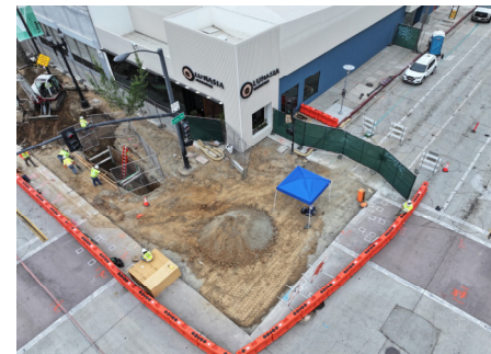
Colorado and Lake Westbound Station Construction
