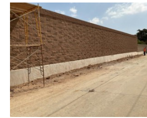
Completion of Soundwall Construction
