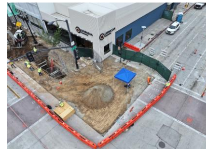
Colorado and Lake Westbound Station Construction
