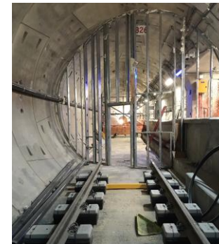
Removal of BR Bulkhead Wall at PLE1 and PLE2 Interface
