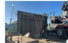
Installing Shear Keys on Abutment 1 at Sepulveda
