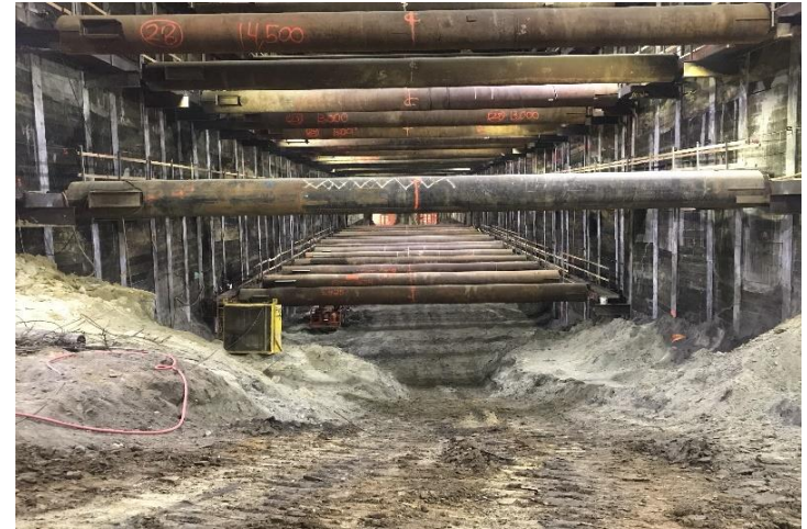
Century City Constellation Station - Excavation Progress
