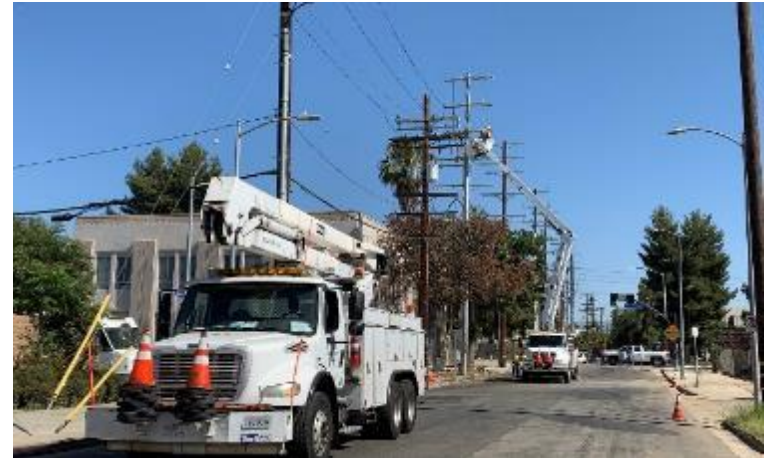
DWP Overhead Construction at Vesper
