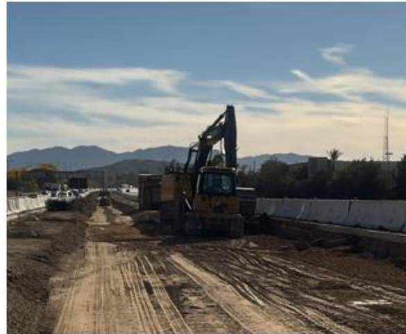
On-Going Roadway Excavation in the Median
