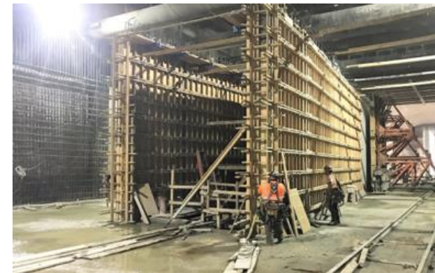
East Interior Wall Formwork at Wilshire/La Cienega
