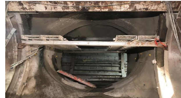
Excavation Complete at Cross Passage #16 (Reach 2)
