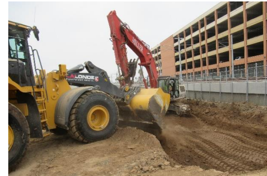
On Site Backfilling Work
