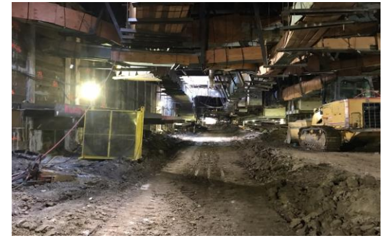
Constellation Station Box Excavation
