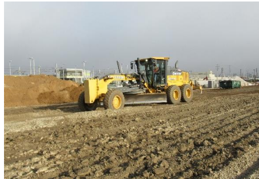
Backfill Work at South End of Site
