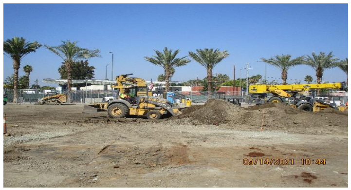
Expo Station – Continue fine grading the entire Park & Ride area.
