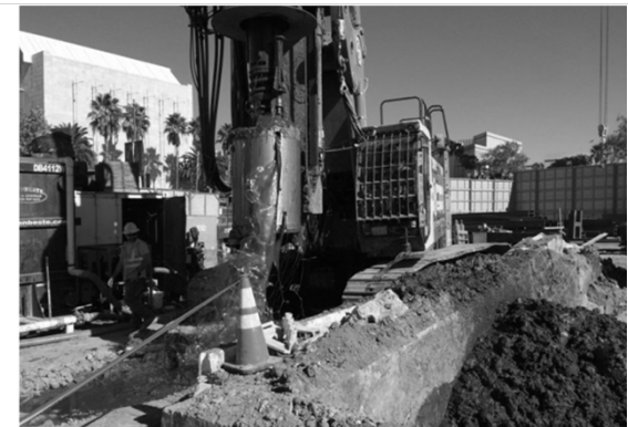
Drilling Piles at Ogden Yard
