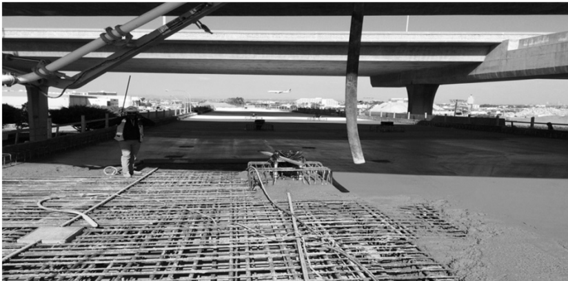
Greenline underpass deck concrete placement in progress
