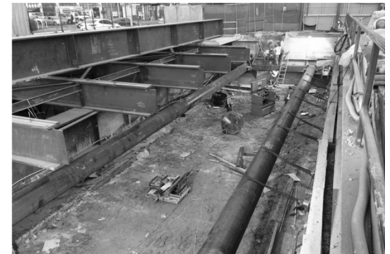
Installing Strut at Wilshire/La Brea Station
