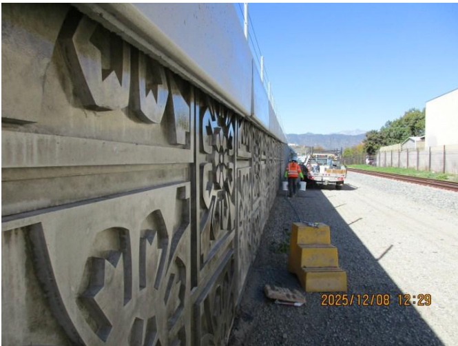
Anti-graffiti coating on the wall along the Metro Train Corridor
