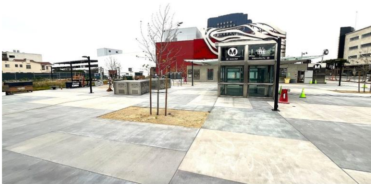
Wilshire/Fairfax Station Plaza Level
