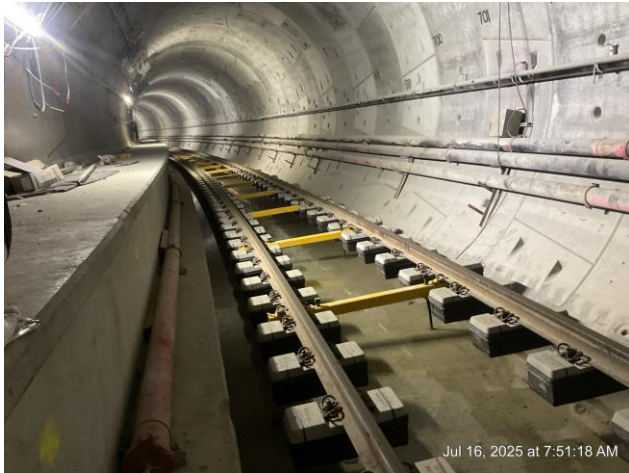
BR Tunnel Reach 5 Track Installation
