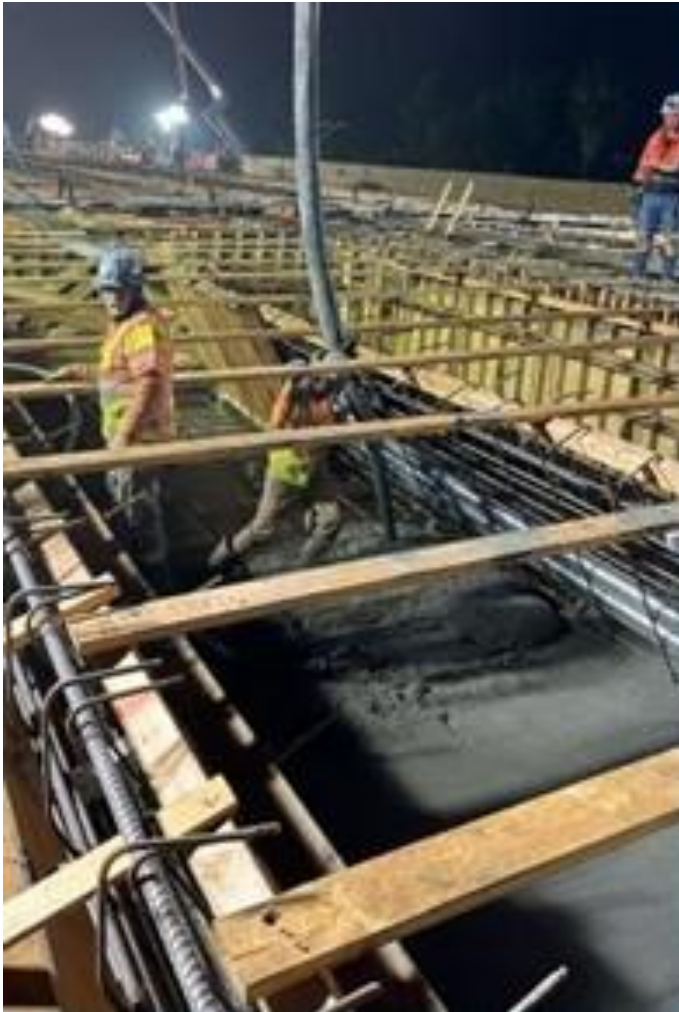
Concrete Placement for Van Nuys Bridge
