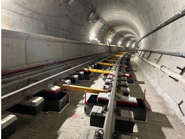
Special Trackwork Double Crossover West of Westwood/VA Hospital Station
