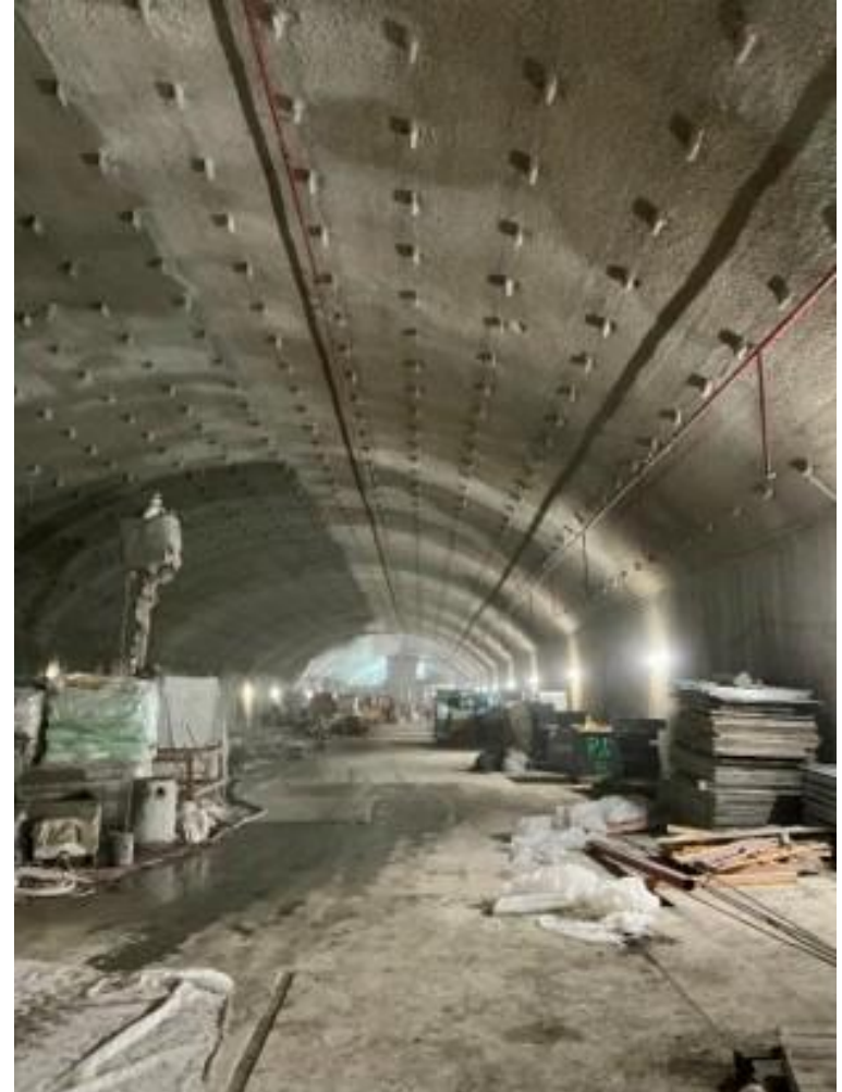
Westwood/VA Hospital Station Arched Roof
