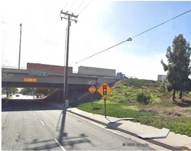
Utilities Relocation at Norwalk Blvd. (North SR-91)
