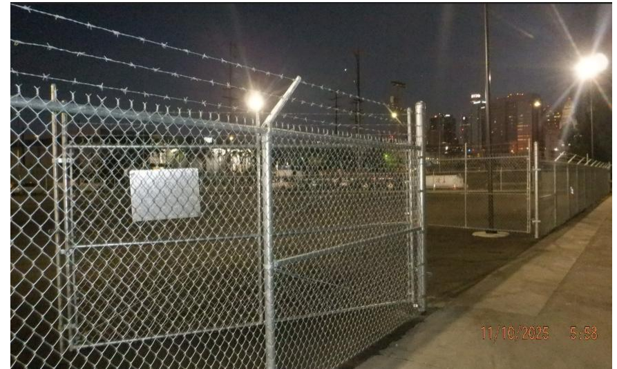
Fencing & site lighting installed (December 2025)
