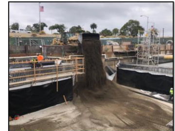
Westwood/VA Hospital Station: Backfilling above the Main Entrance
