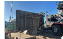
Installing Shear Keys on Abutment 1 at Sepulveda
