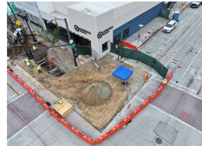
Colorado and Lake Westbound Station Construction
