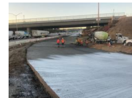
LCB Paving Valencia SB Onramp
