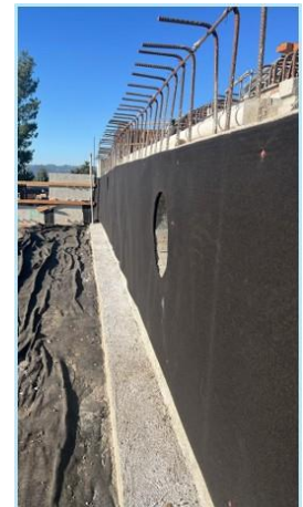
Drain board on Van Nuys Abutment 5 Back Wall
