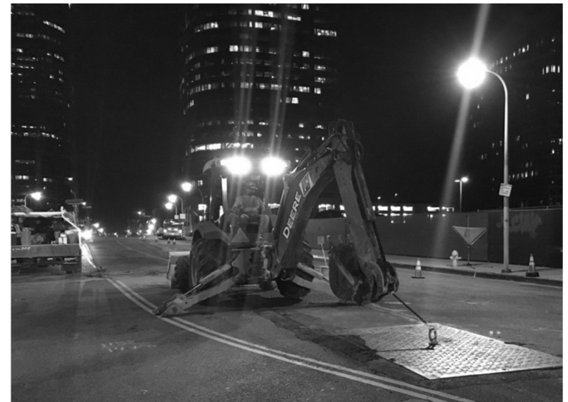
Telecom Joint Trench Construction along Constellation Boulevard
