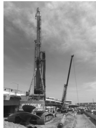
First pile drilling
