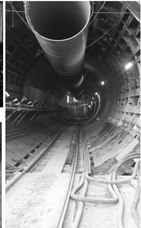
Tunnel entrance at 1 st /Central Station
