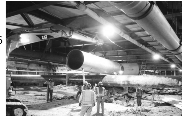
Pipe Strut at Wilshire/La Brea Station
