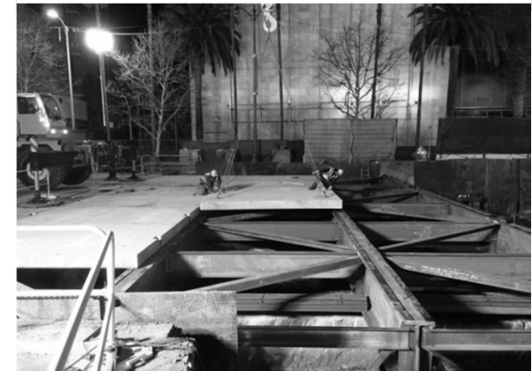
Placement of Deck Panel at Wilshire/Fairfax
