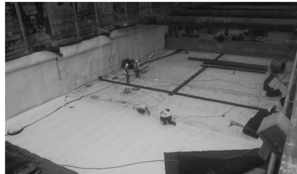
HDPE placement at 2 nd /Hope Station
