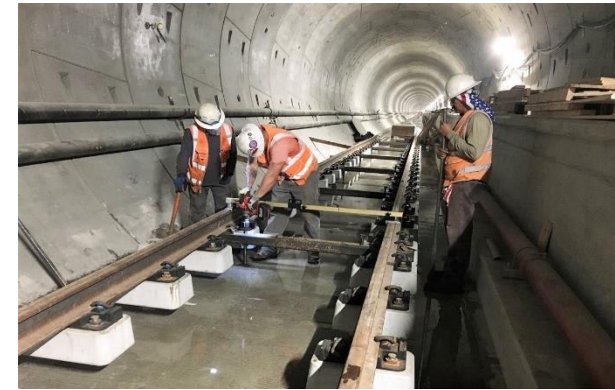
Reach 1 North Tunnel Trackwork Installation
