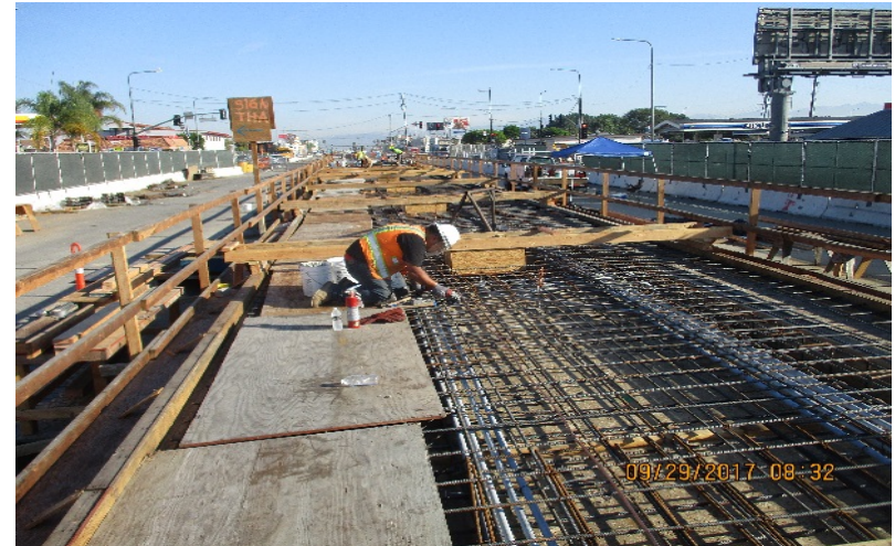
Installing components for platform deck at Hyde Park Station
