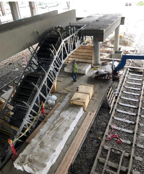
Escalator and platform work @ Mezzanine
