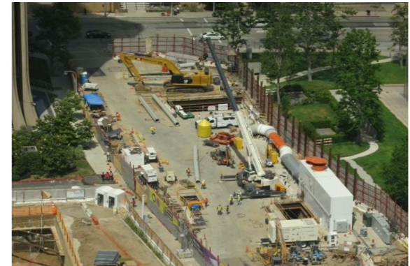
TBM Launch Box Overview in Century City
