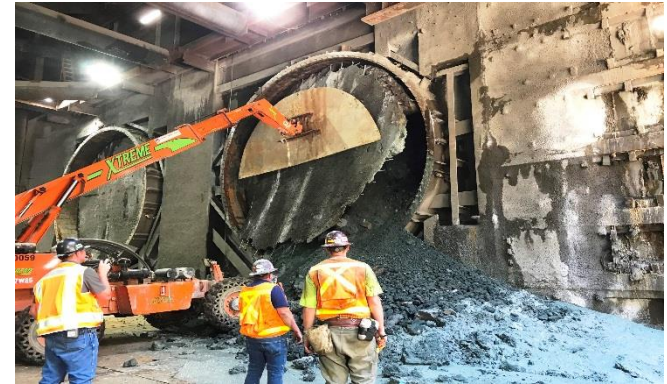
TBM #1 Break Through at Wilshire/Western
