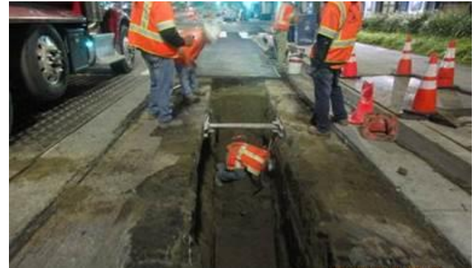
Installing Riser for Water Pressure Test
