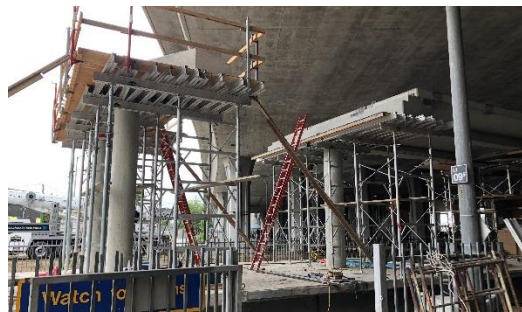
Formwork @ Blue Line Platform/Mezzanine
