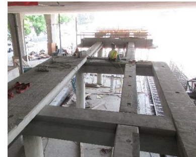
Precast @ Blue Line Mezzanine Extension
