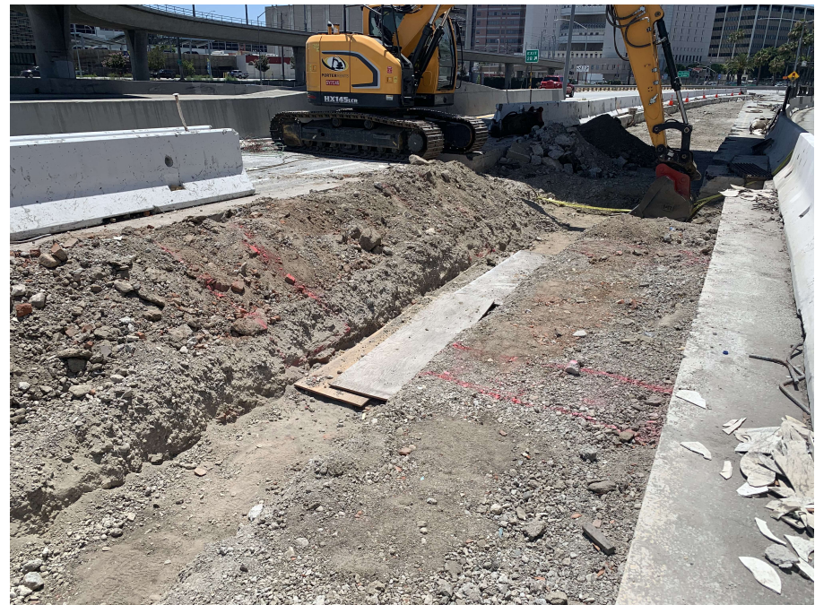
Archaeological Data Recovery Begins at Storm Drain
