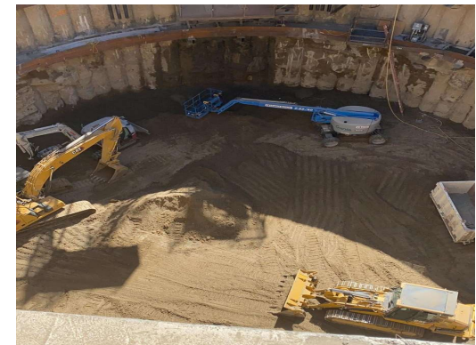
TBM Launch Shaft Excavation
