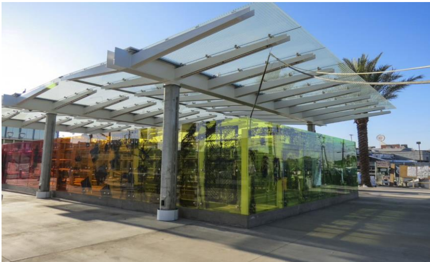
LEIMERT PARK STATION – Main entrance canopy art installation
