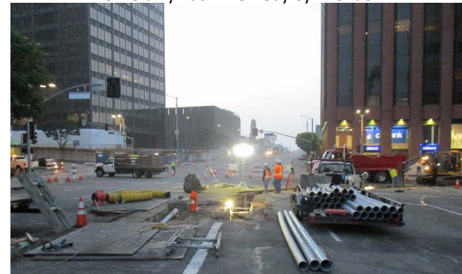
Power Conduit Installation at Wilshire and Westwood Boulevards
