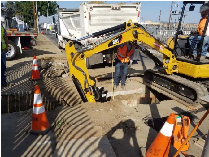
UG conduits crossing the street
