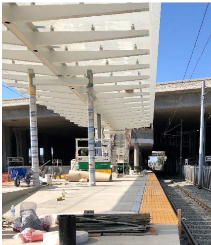
Blue Line Platform Work
