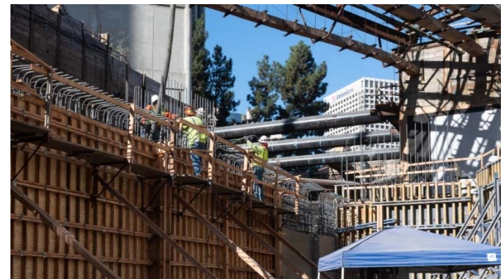
Setting wall forms at Grand Av Arts/Bunker Hill Station
