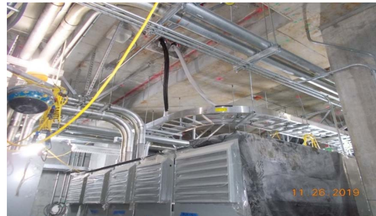
Auxiliary power high voltage cable tray in Martin Luther King Jr. Station
