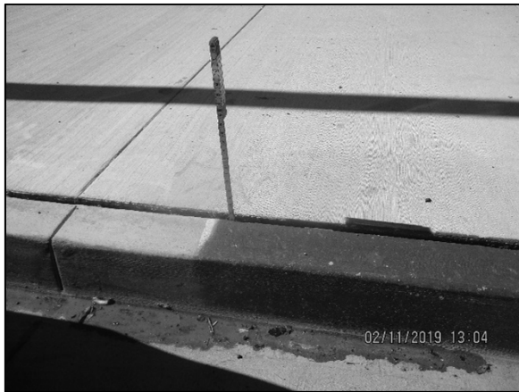
Heaving of Sidewalk (West side, 54 th & 57 th )
