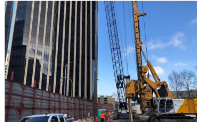
Soldier Pile Installation in Century City
