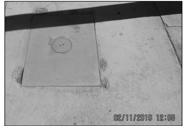
Spalling at Meter Box (West side, 50 th & 52 nd )
