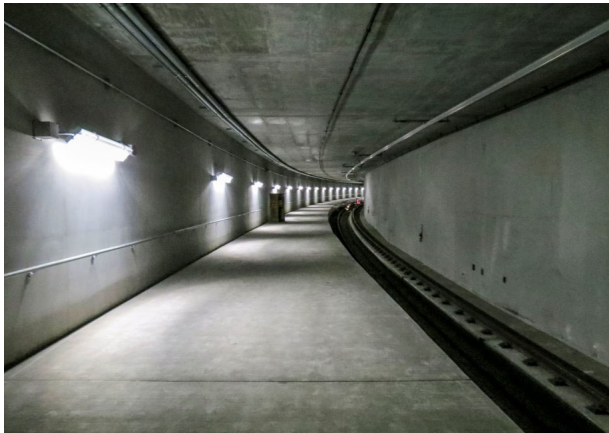
LEIMERT PARK STATION – Train tunnel with emergency walkway
