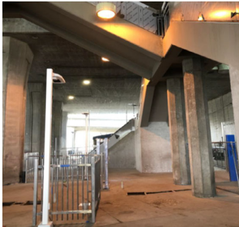
Completed concrete work @ C Line west
