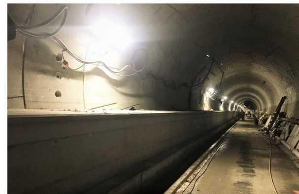
Reach 1 Tunnel Invert & Walkway Concrete Placement
