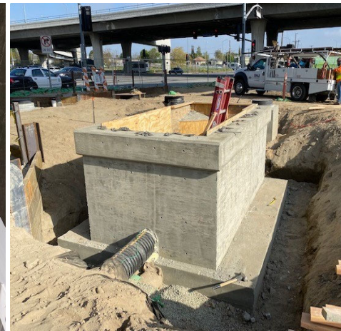
Formed & poured North Drainage System
