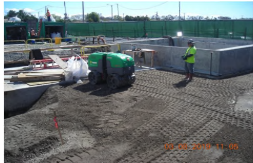
Back filling/compaction of Expo/Crenshaw Station Plaza
