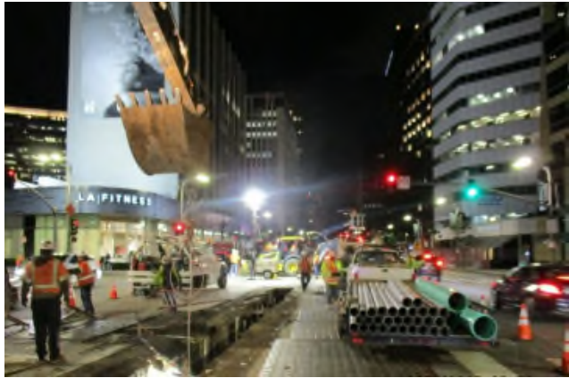
LADWP Water Pipe, Valve and T-Section Installation
