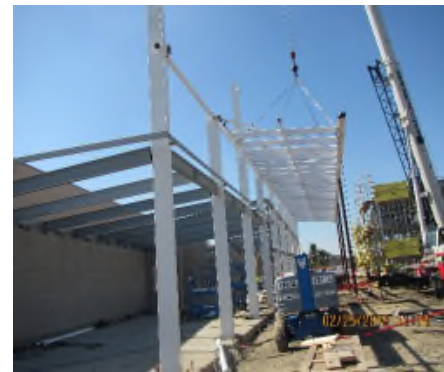
Structural Steel Installation for Mobility Hub
