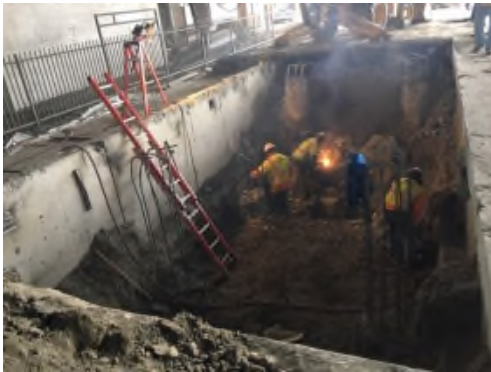
Demolition of Rail Platform
