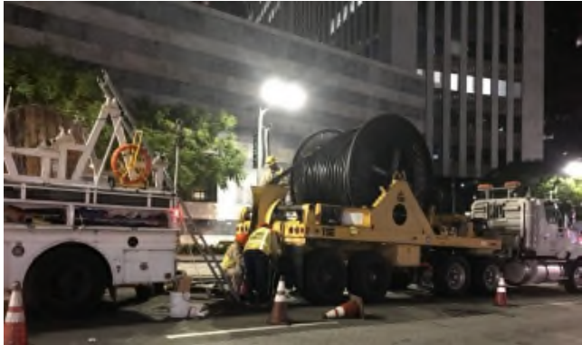
LADWP Cable Pulling
