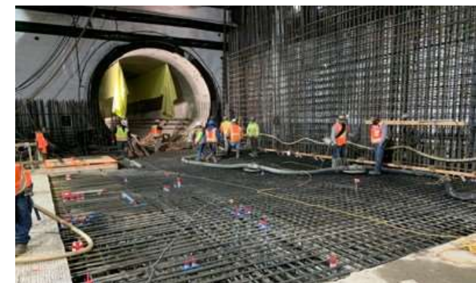
Concrete Placement at Wilshire/La Cienega Station (West)
