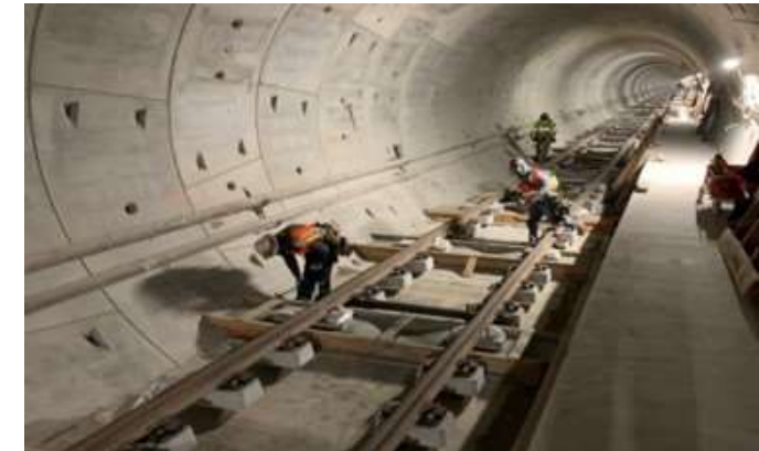
Reach 1 North Tunnel Trackwork Installation
