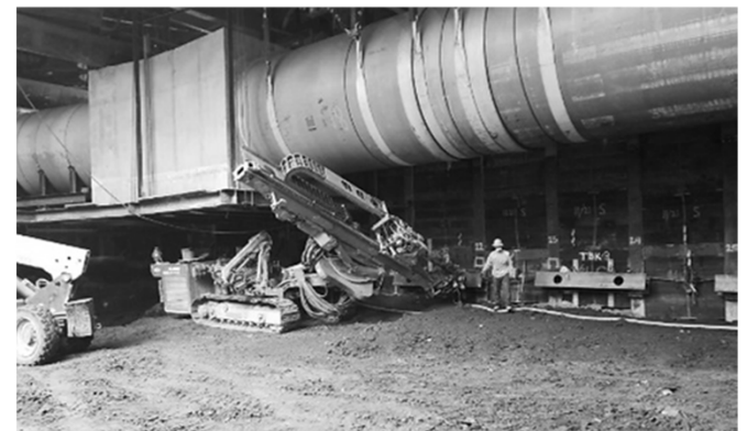
Tieback installation at Historic Broadway Station
