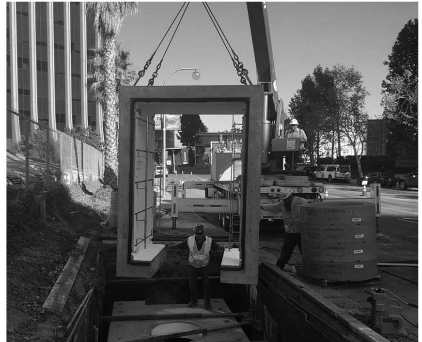
AT&T CA manhole Installation in Century City
