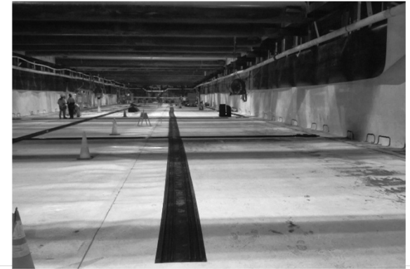
Wilshire/La Brea Station
