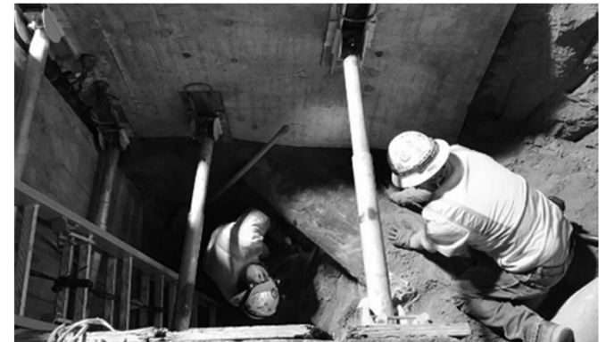
Excavation of 20" waterline on Central Avenue
