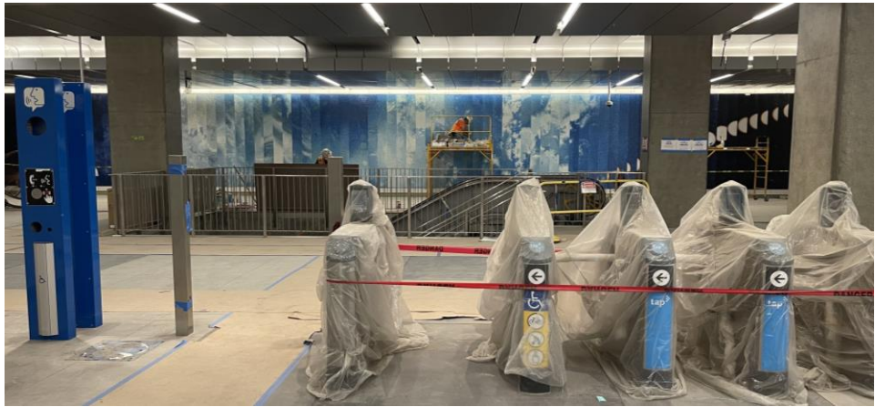
Expo/Crenshaw Station – Artwork installation and fare gate equipment
