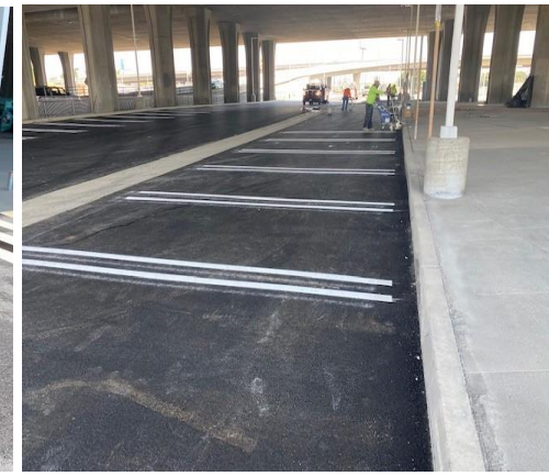
Park & Ride Lot completed
