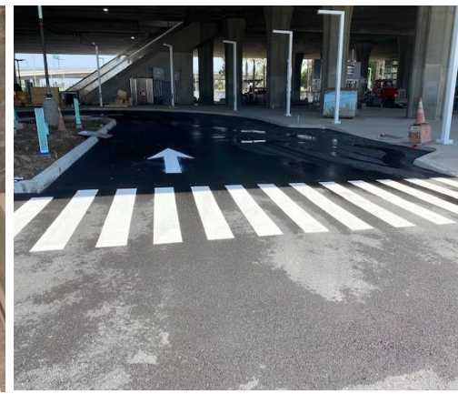
Passenger Pick-up & Drop-off area completed
