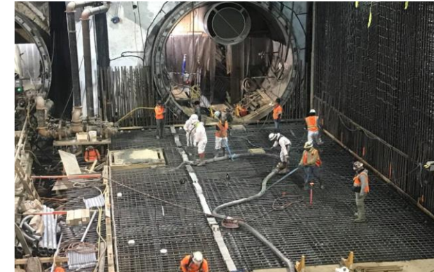
Wilshire/La Brea West Hammerhead Concrete Placement
