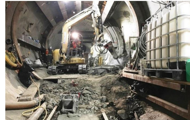
Work at Cross Passage #12
