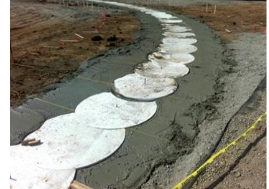
First 100 ft. of TTES Guide Wall Placement at Western VA Staging Area
