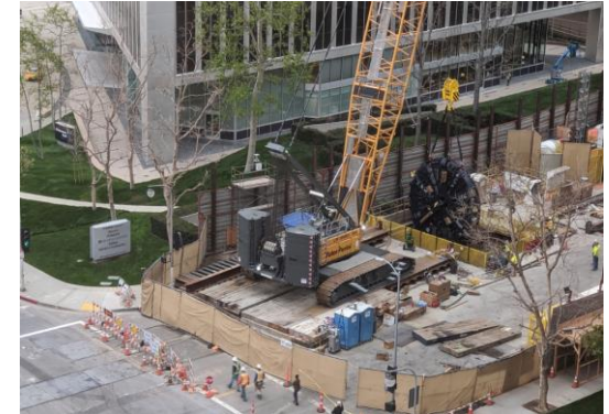
Lowering of TBM Cutterhead at the Launch Box in Century City
