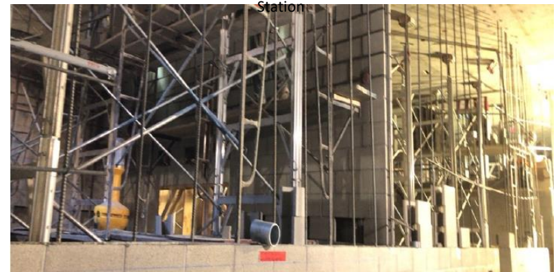
Conduit installation at CMU walls
