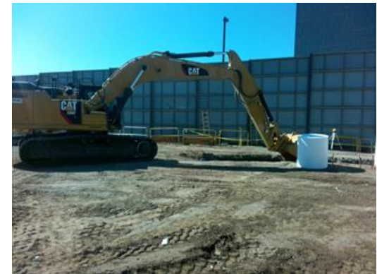
Excavation of TTES Guide Wall Trench
