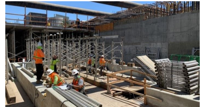
Aluminum shoring installation for roof deck the future Little Tokyo/Arts District Station
