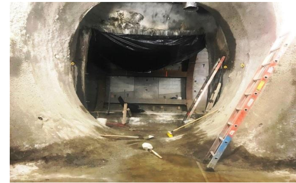
View of Reach 1 Cross Passage #8
