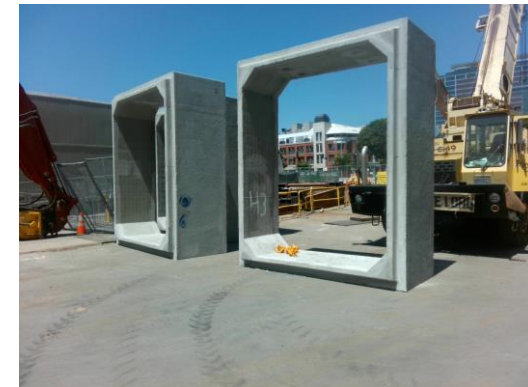
Reinforced Concrete Boxes for Storm Drain Relocation
