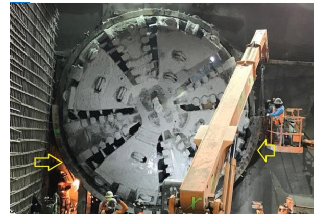
Purple TBM Arrival of Wilshire/La Cienega Station
