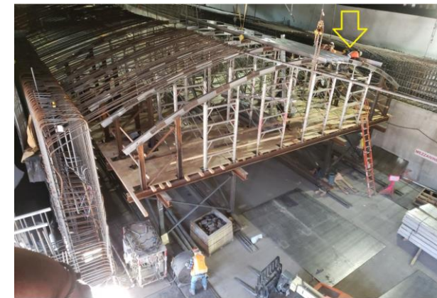
Installing Roof Falsework at Wilshire/Fairfax Station
