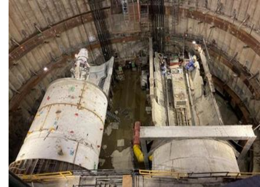
TBM Assembly Overview at Tail Track Exit Shaft
