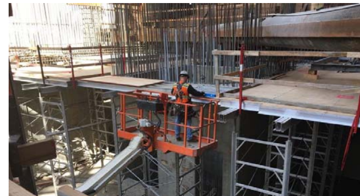
Concourse level concrete pour prep at Grand Ave Arts/Bunker Hill Station
