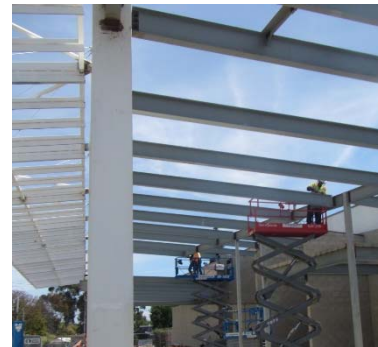
Structural Steel Installation for Mobility Hub
