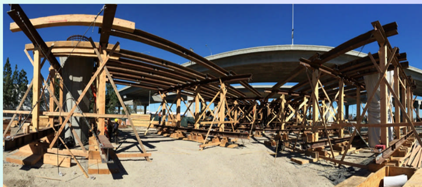
Crenshaw tie-in with Green line falsework construction
