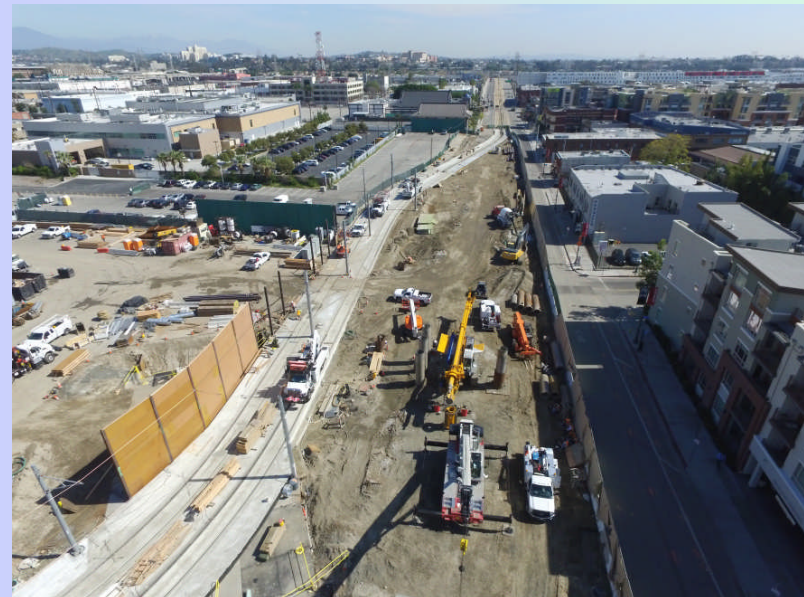
Shoofly installation at 1 st Street
