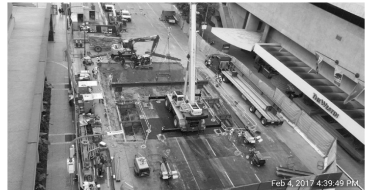
Installation of deck beams on Flower Street
