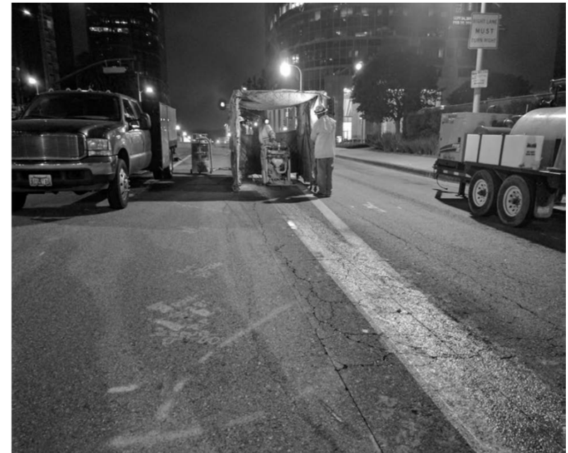
Telecom Joint Trench Construction along Constellation Boulevard
