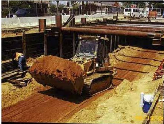
Figure 4-13: Track Loader beneath Struts
