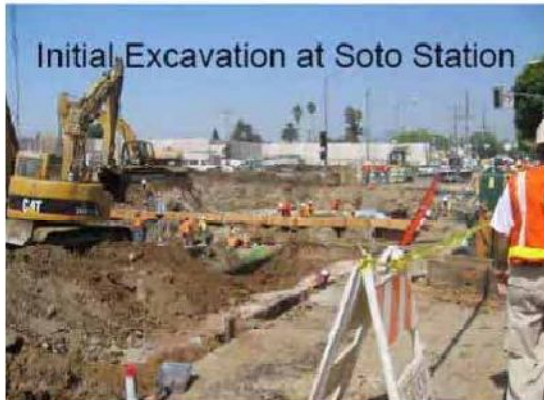
Figure 3-2: Initial Excavation at Soto Station
