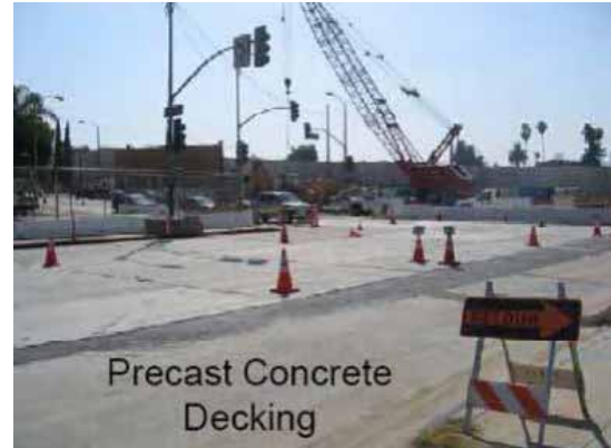
Figure 3-3: Precast Concrete Decking
