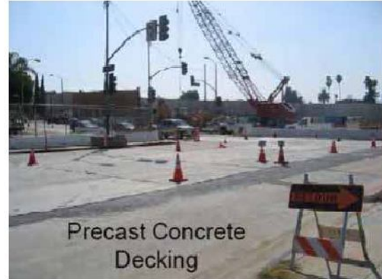
Figure 3-3: Precast Concrete Decking
