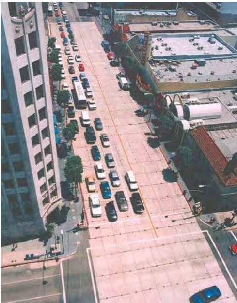
Figure 3-1: Roadway Operations Restored on Temporary Decking System
