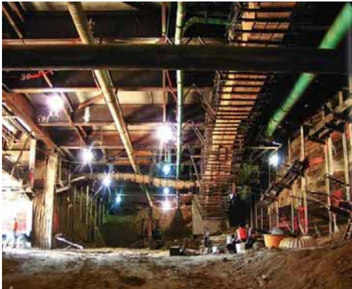
Figure 3-17: Utilities Hung from Deck Beams
