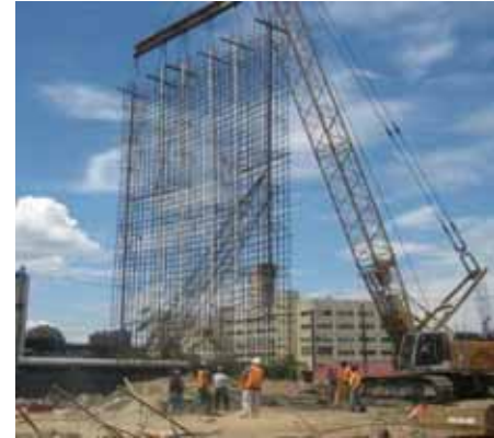
Figure 3-13: Steel Reinforcement Cage for Slurry Wall
