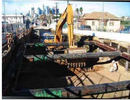
Figure 4-12: Hydraulic Excavator between Struts
