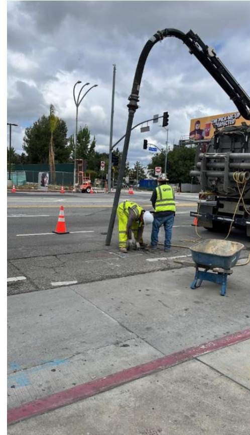
Potholing at Van Nuys Blvd
