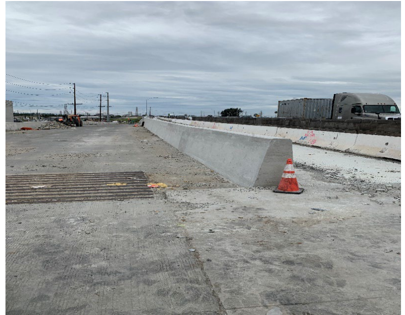
NB Crenshaw Blvd to SB 405 on ramp (RW#803) completed concrete barrier slab (Looking North)
