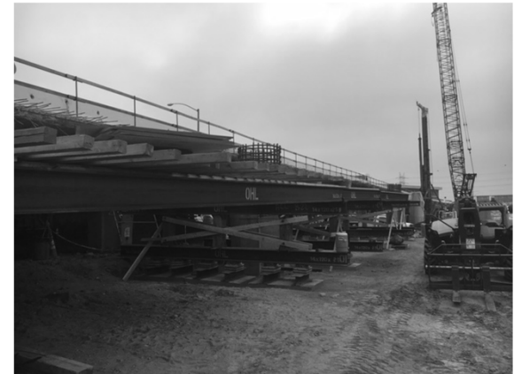
False work on south side
