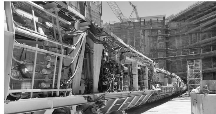
TBM in Grand Av Arts/Bunker Hill Station preparing for relaunch
