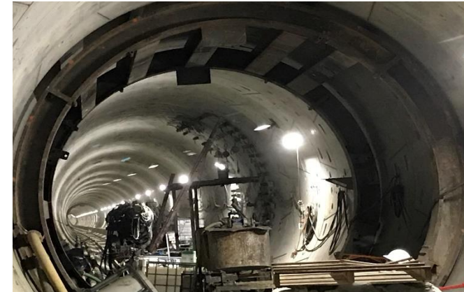
Reach 2 Cross-Passage Excavation Preparation
