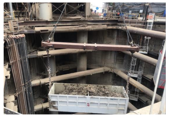
Tunnel Muck Removal in Century City
