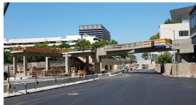
Asphalt pavement complete along Hope Street
