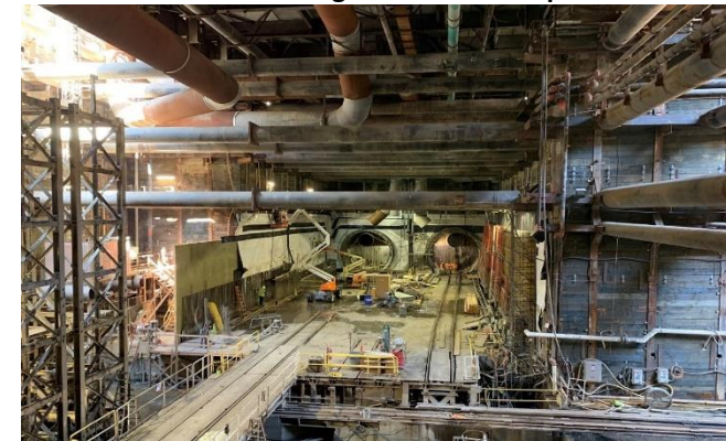
Track Level View of Wilshire/La Brea Station
