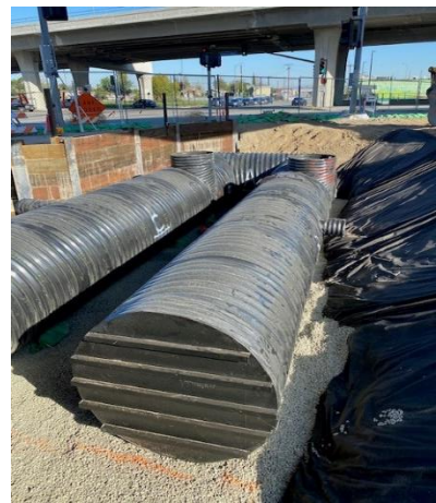
Installed cistern for North GSRD
