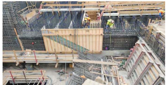
Formwork and cleaning at Historic Broadway Station
