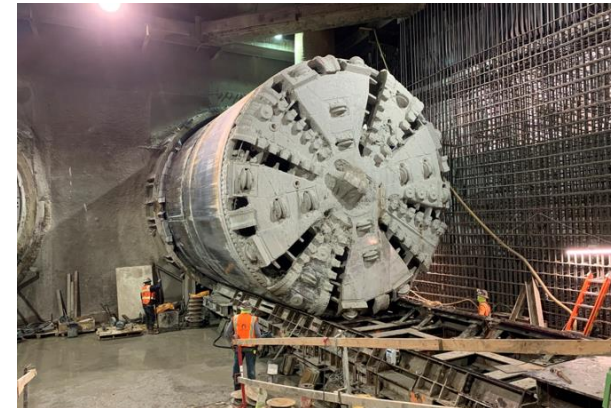
Red TBM Arrival of Wilshire/La Cienega Station
