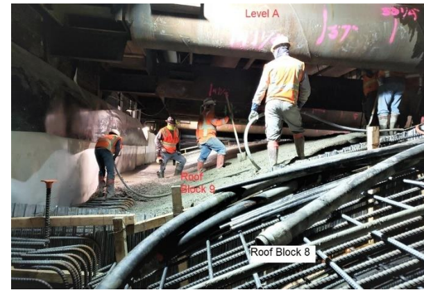
First Roof Concrete Placement at Wilshire/Fairfax Station
