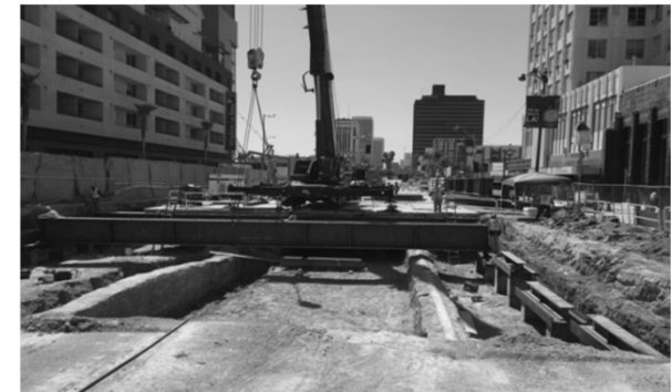
Installation of deck beams at Wilshire/La Brea Station
