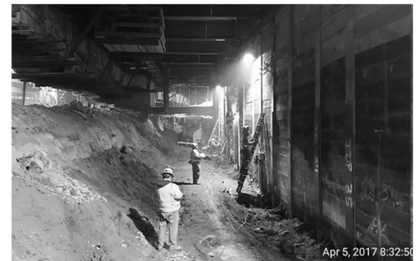
Excavation and utility hanging under 2 nd Street
