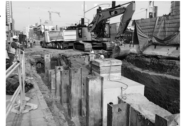
Decking Operation at Wilshire/Fairfax Station
