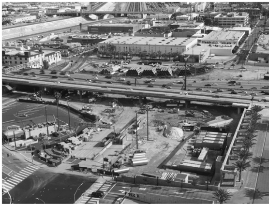
Aerial view of site
