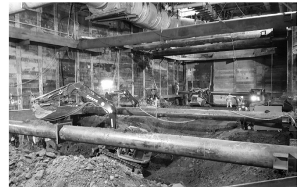
Excavation and lagging for TBM Retrieval Shaft
