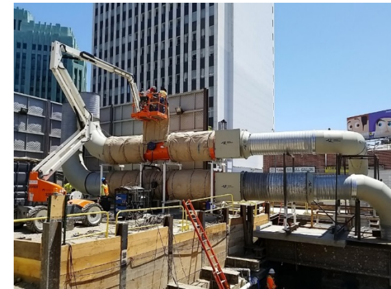
Wilshire/Western Retrieval Shaft
